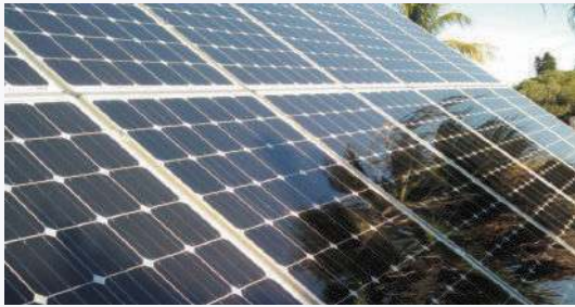
Figure 47: Tree grows adjacent to your PV system and casts its shadow on modules
