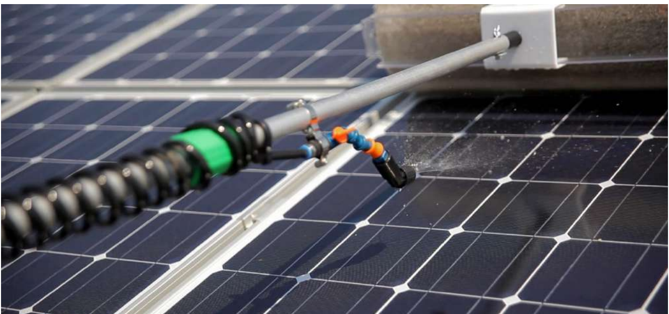
Figure 45: Wet cleaning using an automated system
