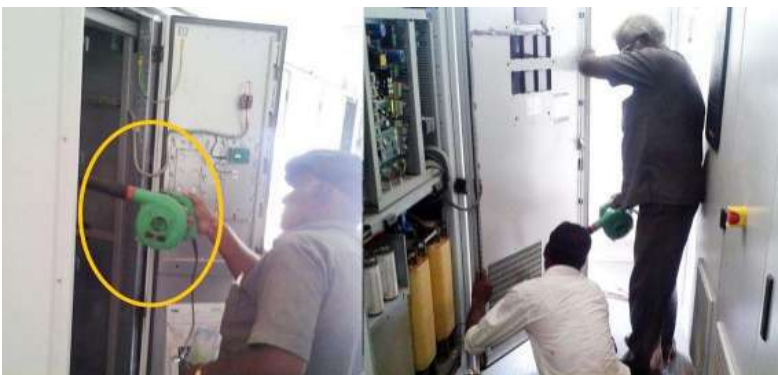
Figure 89: Cleaning inverter using blower
