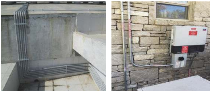
Figure 101: Proper cable routing
