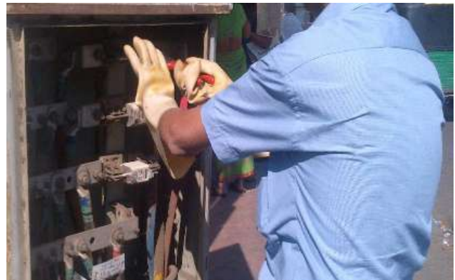
Figure 159: Correct practice - With safety gloves
