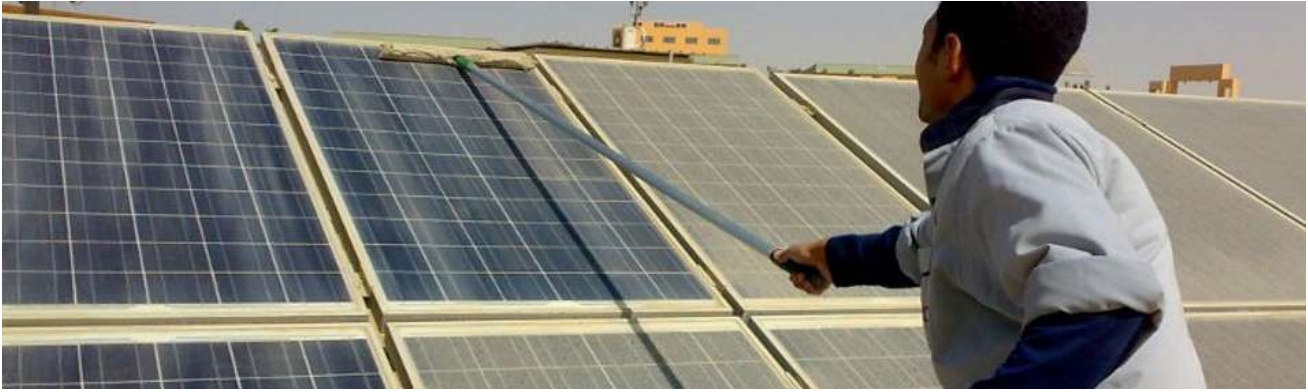
Figure 42: Dry Cleaning Method (Manual)
