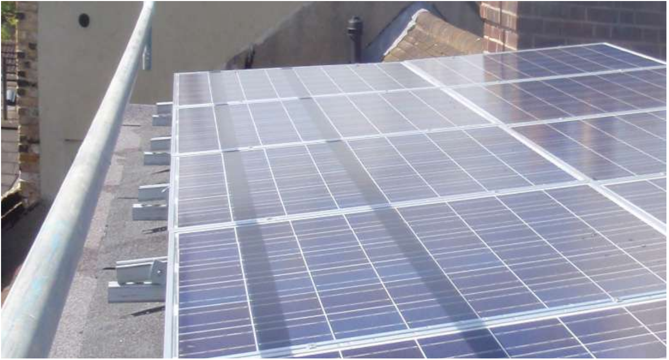
Figure 51: Shading due to nearby poles on terrace
