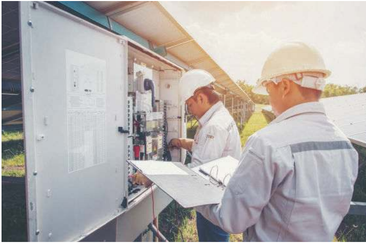
Figure 94: Written inspection report of Inverter
