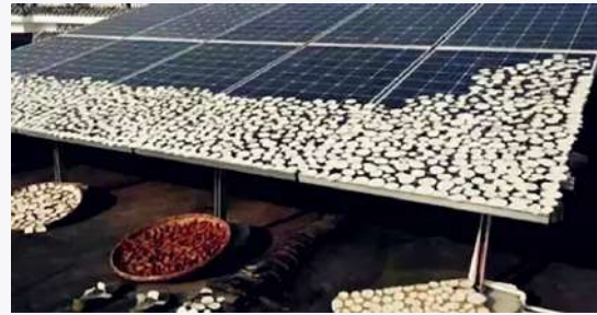
Figure 50: Shading due to drying crops
