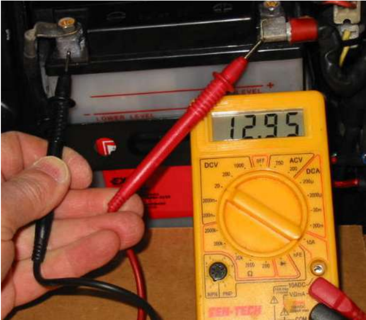
Figure 147: Battery Load test using Multimeter
