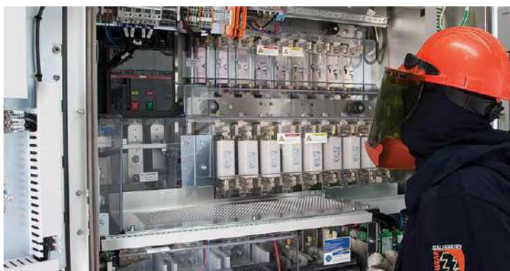
Figure 92: Check inverter fuses
