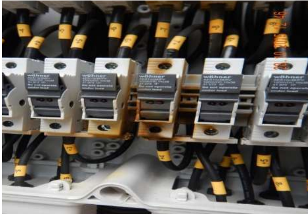
Figure 120: Fuses - Burnt out
