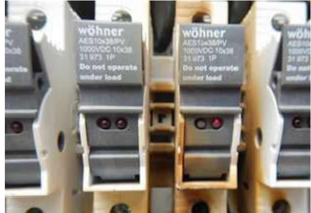
Figure 120: Fuses - Burnt out
