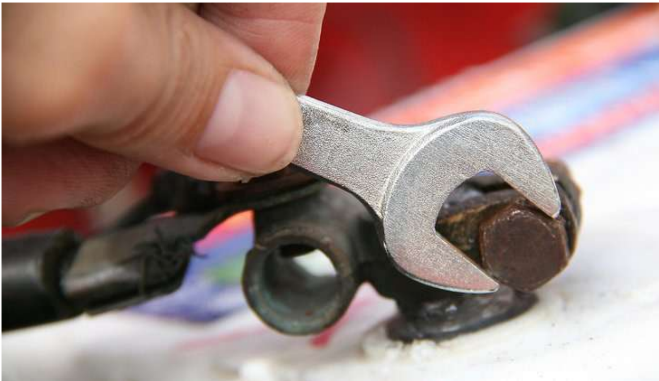
Figure 131: Tightened battery terminals
