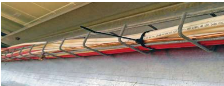
Figure 113: Cables are tied using cable tie
