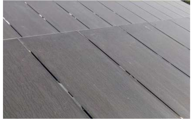
Figure 24: Cleaning Required Shortly (No significant financial impact)
