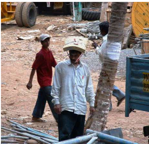
Figure 150: Incorrect practice - Without safety helmet
