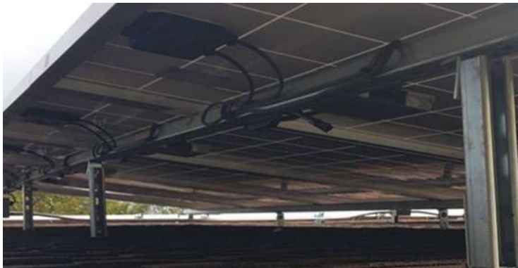
Figure 104: Correct cabling connection
