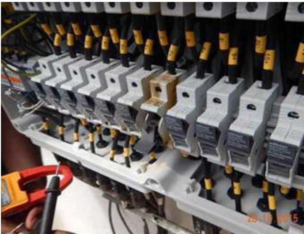
Figure140: Testing using clamp meter
