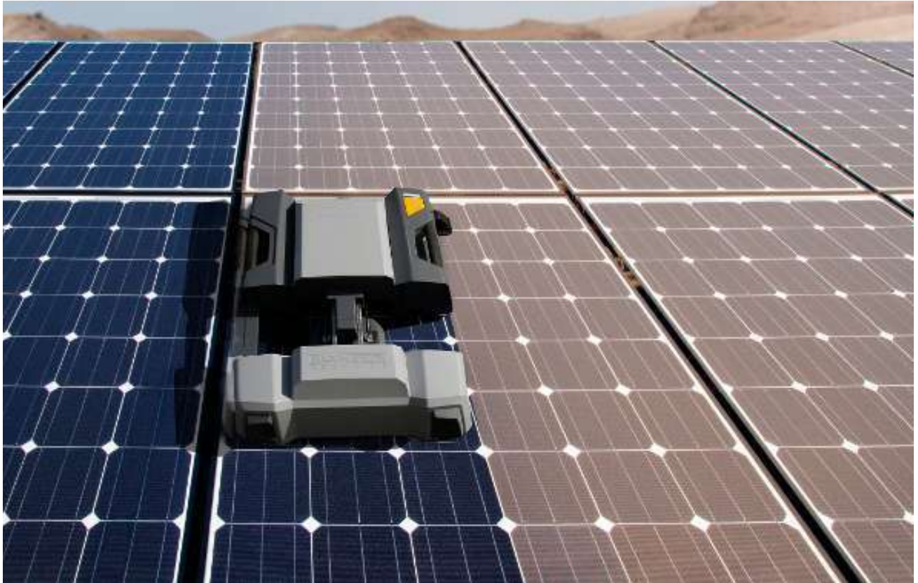
Figure 46: Dry cleaning method using an automated system
