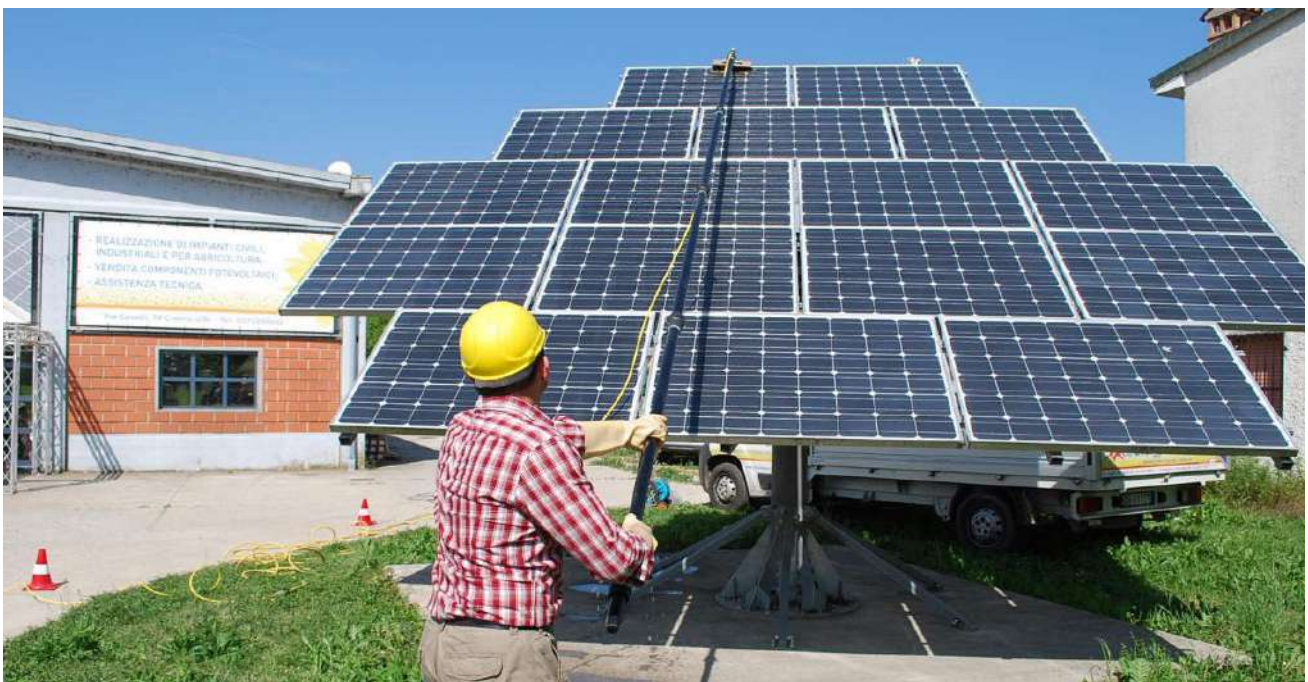
Figure 37: Wet Cleaning (Manual)
