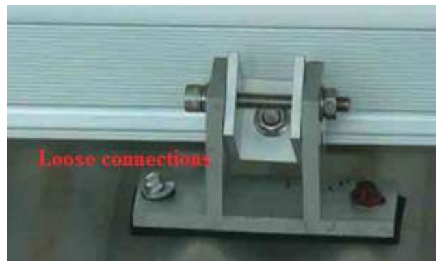
Figure 118: Loosed clamps
